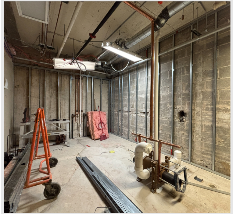
A look at the Lower-Level Restroom with the carrier set for new toilets and in-wall piping set for new sinks. Wall framing is in progress!
