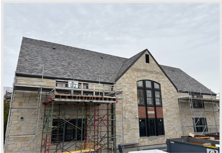
Scaffold installation in progress on the east side of the building, getting prepared for the final existing roof tear-off for the project!
